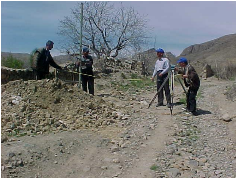
Picture 57. Geodesy-measurement work is performed on the ancient ganat wells
