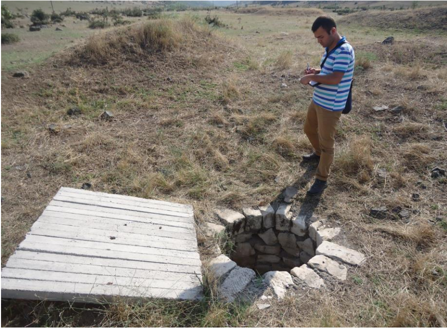
Picture 80. The ganat well part on the surface.
