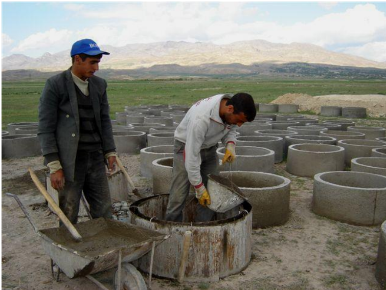
Picture 61. Concrete rings preparing for the wells. (Nakhchivan)
