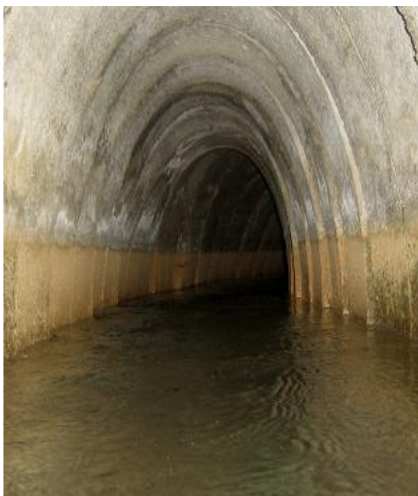
Picture 59. Lineage of the concrete rings put in the ganat bloomer
